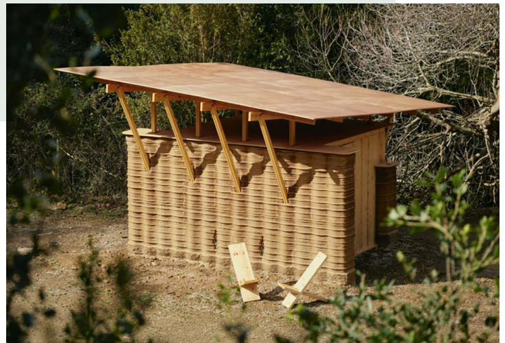
Figure 5 Tova, 3d-printed Earth Architecture, IAAC - Annex A, Case study 003, image: Gregori Civera
