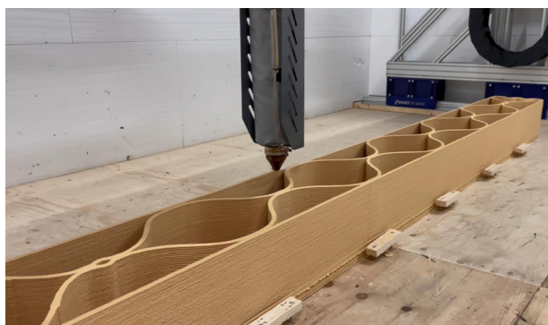
Figure 16 Wohn Homes - Annex A, Case study 014, Image courtesy of Wohn Homes
