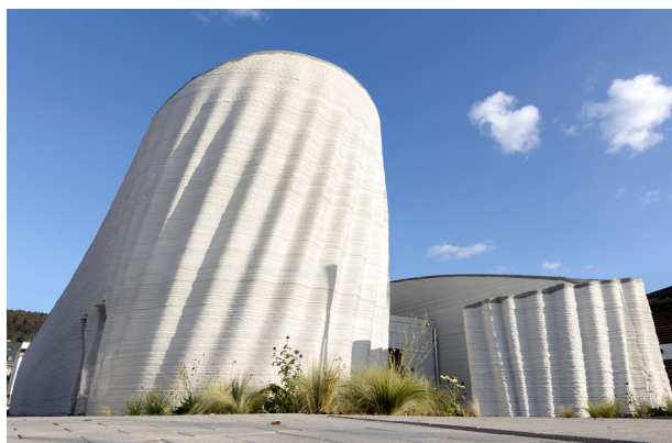
Figure 12: The Wave House Data Center – The first and globally largest
